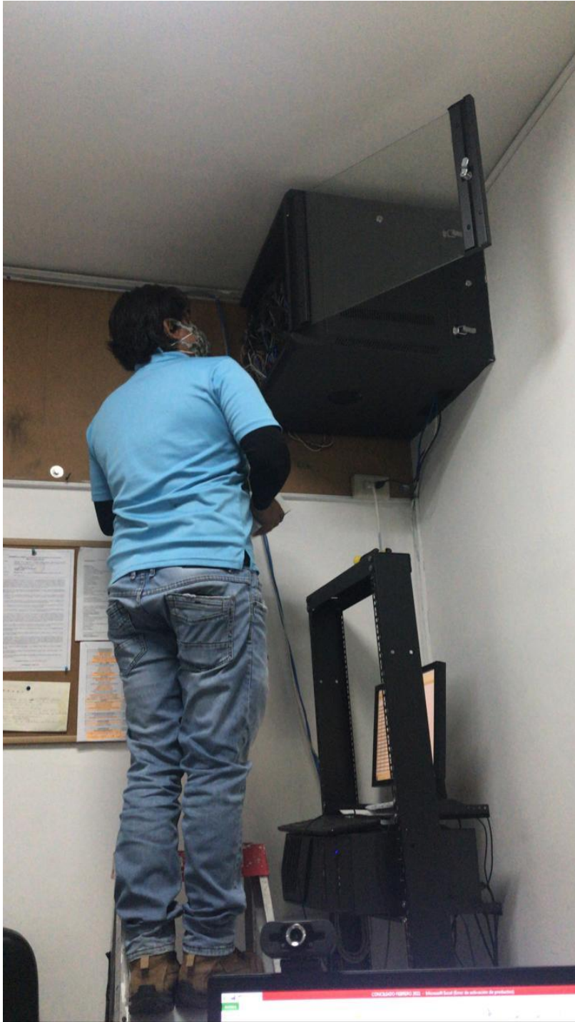
Reparacion del circuito cerrado de television torre 2
